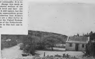
Sturdy concrete homes dot nearly all parts of the island's "Cunucu" or rural districts.
